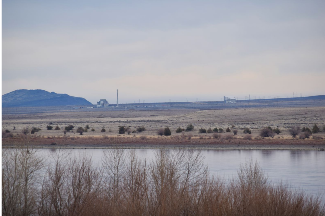
Hanford facilities seen off in the far distance- speculated to be the remnants of one of the larger reactors.
