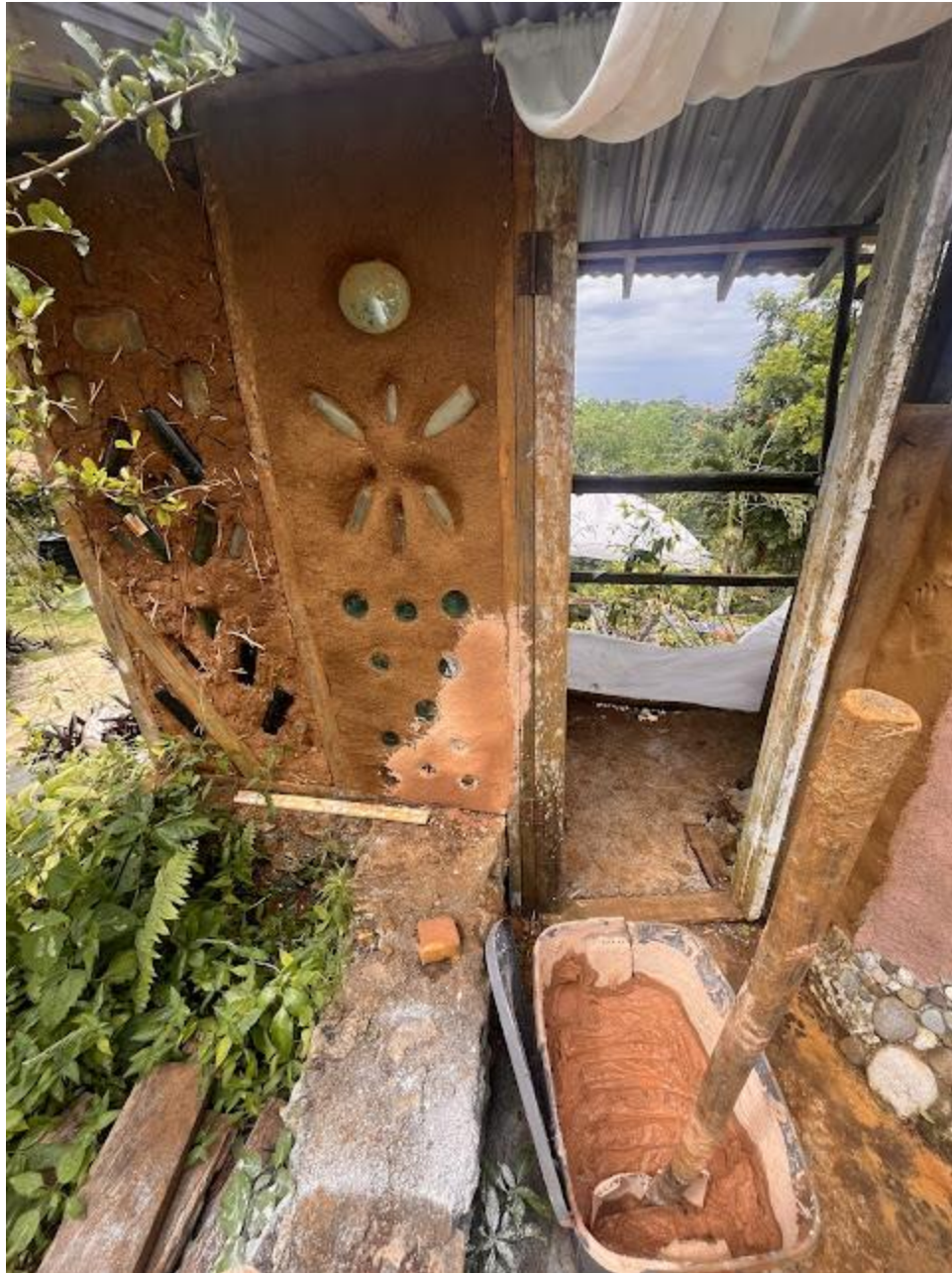
Cob Walls of Compost Outhouse Being Plastered
