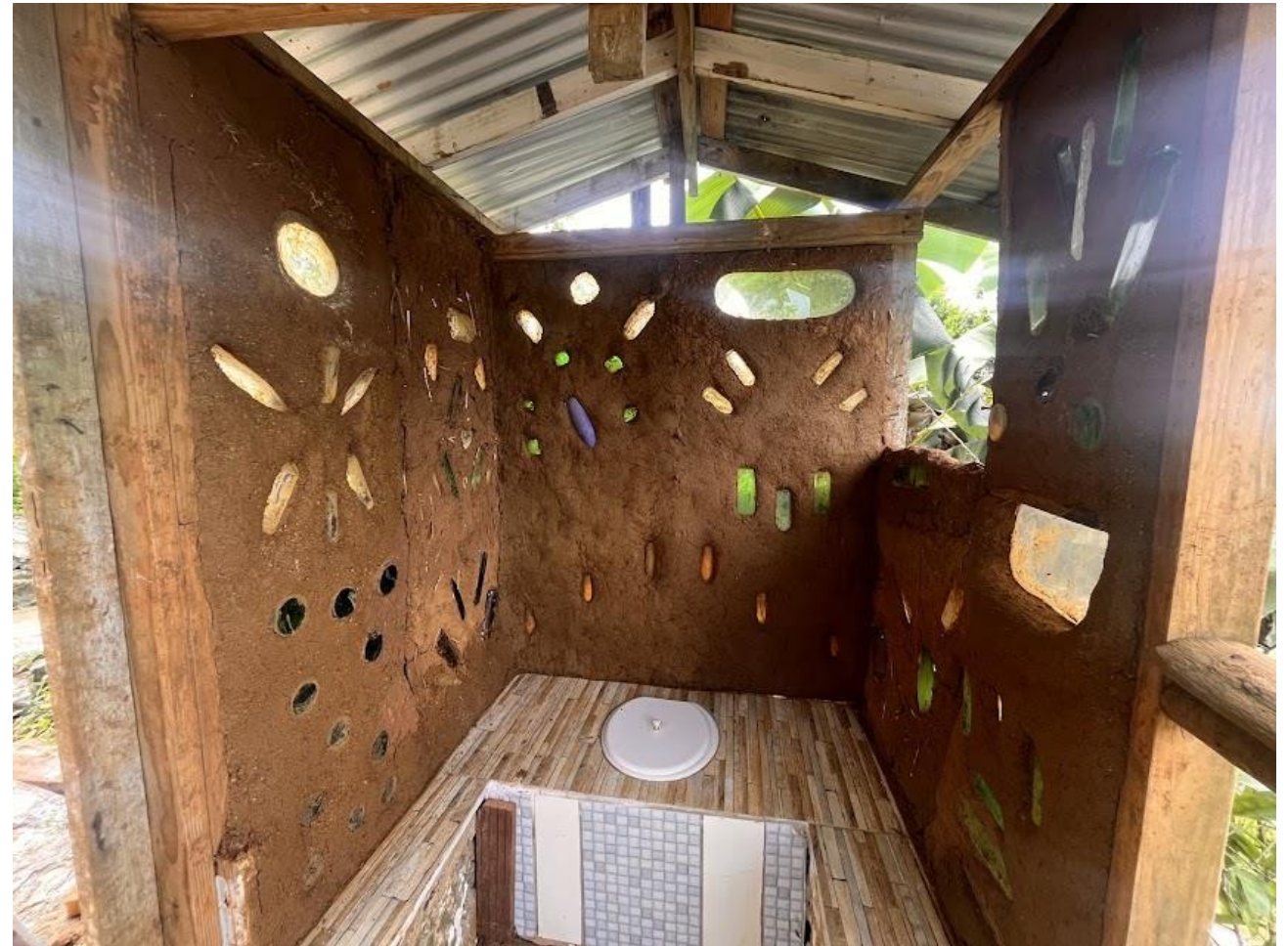
Cob Walls Being Rebuilt
